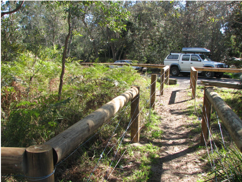
Photo; Heavy duty dune fencing installed at the Etta Road entrance
